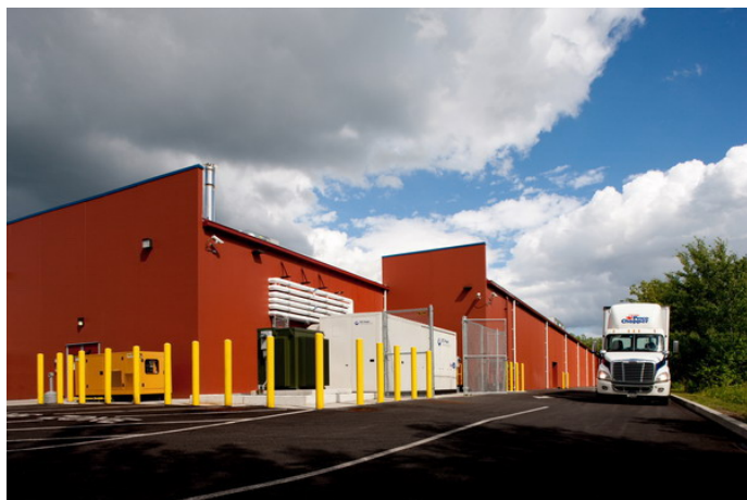
A 400-kW fuel cell (grey box) meets 85 percent of the energy needs of this Price Chopper supermarket in Albany. The installation reduces the building's carbon footprint by 71 tons, provides energy security for perishable items, and saves more than 4 million gallons of water each year. (Photo courtesy of UTC Power)
